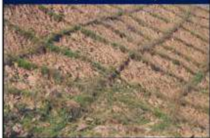
Sodding (checkerboard style)
